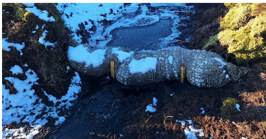
Sheep fleece being used instead of imported coconut coir roll as drain blocking material in peatland restoration work
