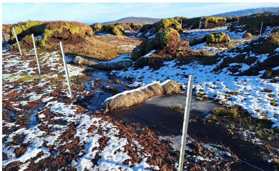
Sheep fleece being used instead of imported coconut coir roll as drain blocking material in peatland restoration work
