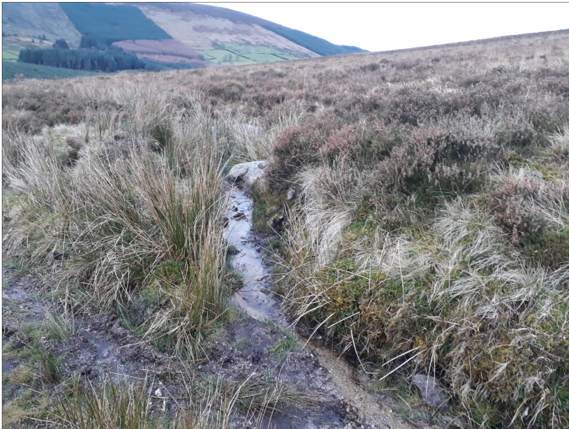
Plate 1. Shores allowing the water to escape off the track.
