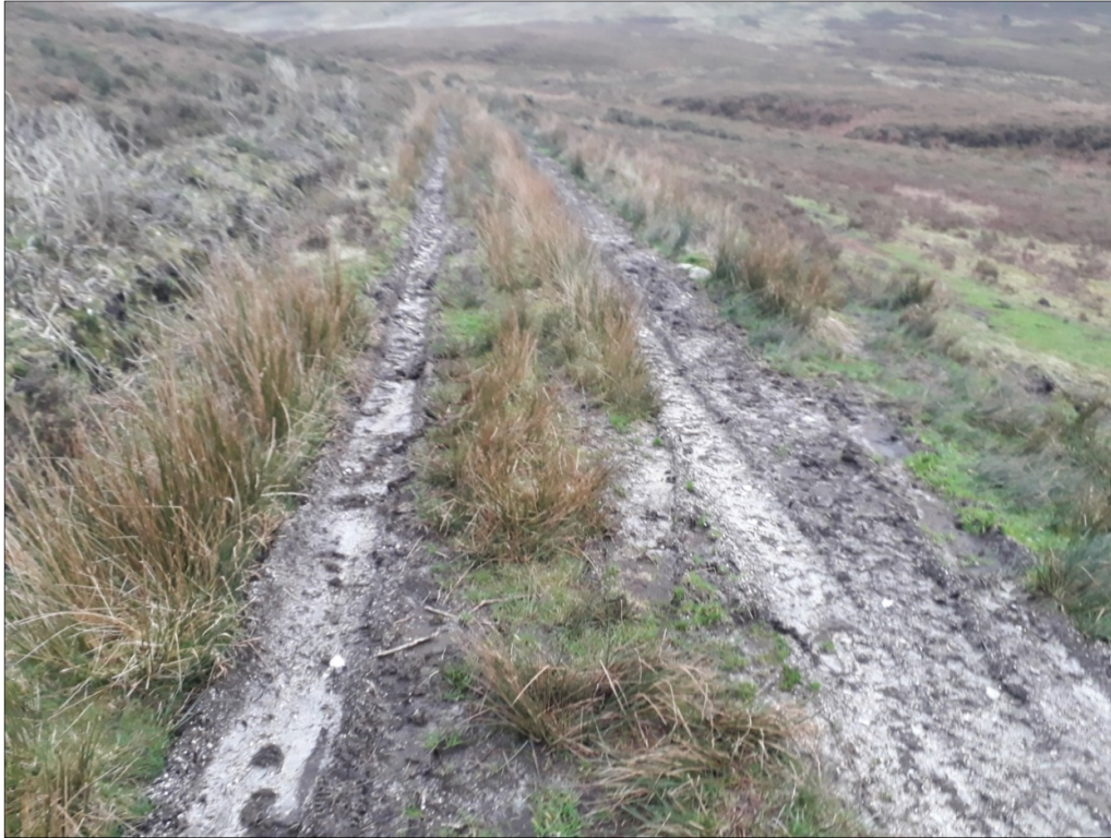
Plate 2. Tyre tracks have created deep channels for water to flow down on the track above the old borrow pit.
