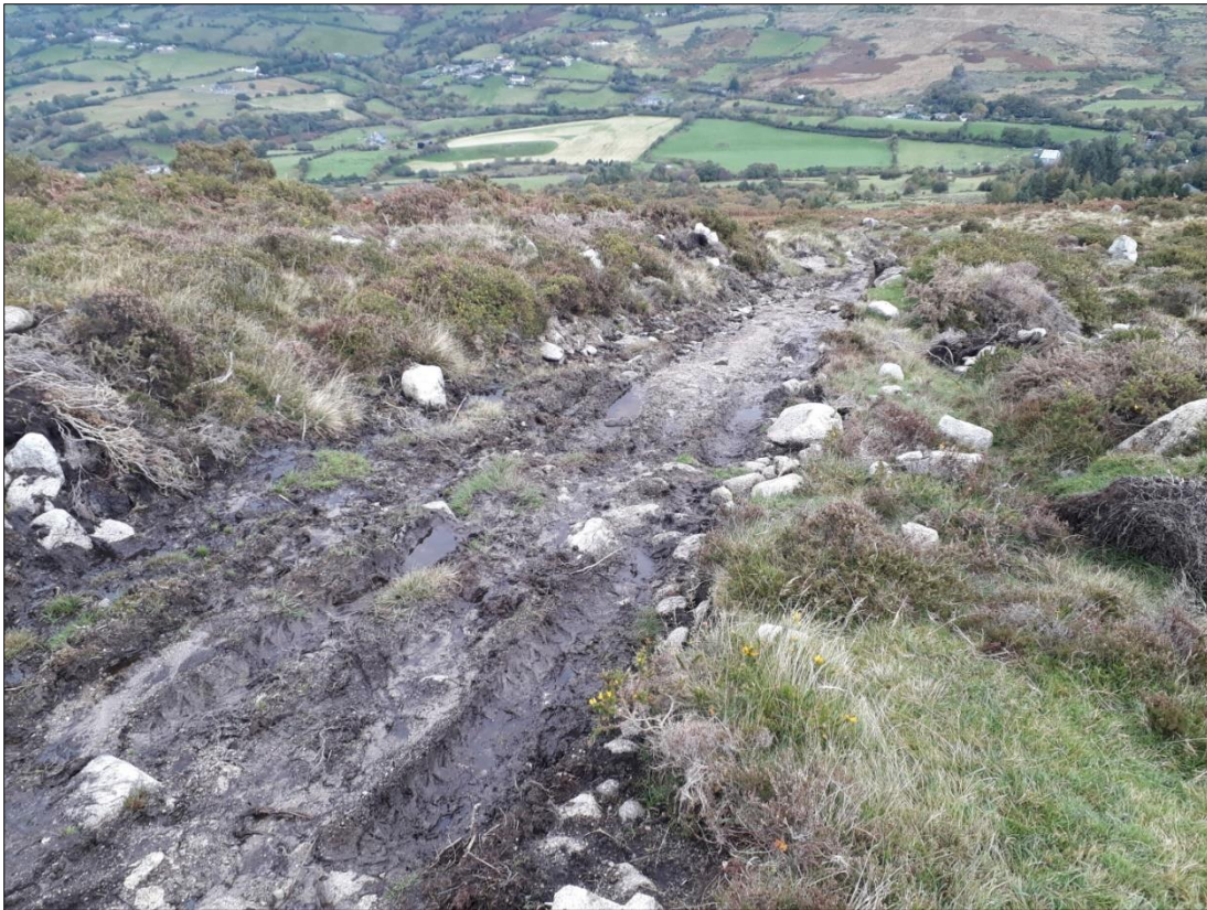
Plate 10. Damage caused by the new section of track.
