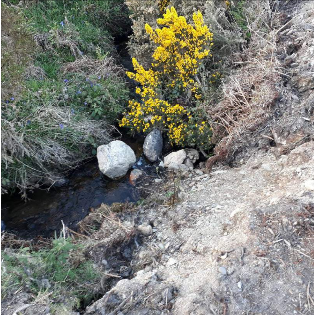
Excavated material and dislodged boulders have entered the watercourse.
