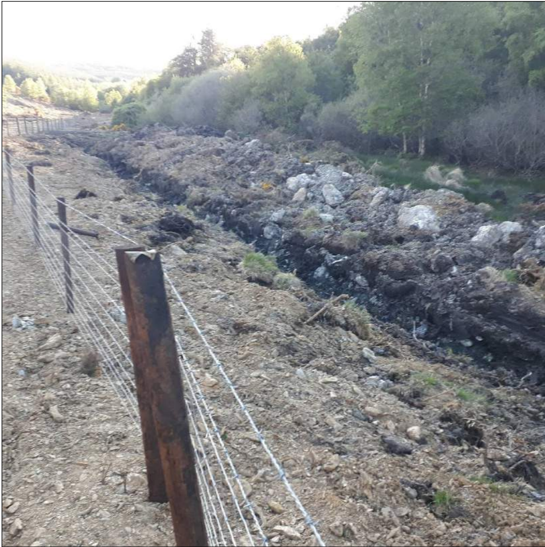
The natural floodplain of the river has been completely destroyed through vegetation clearance, disturbance and drainage with subsequent hydrological and water quality impacts.
