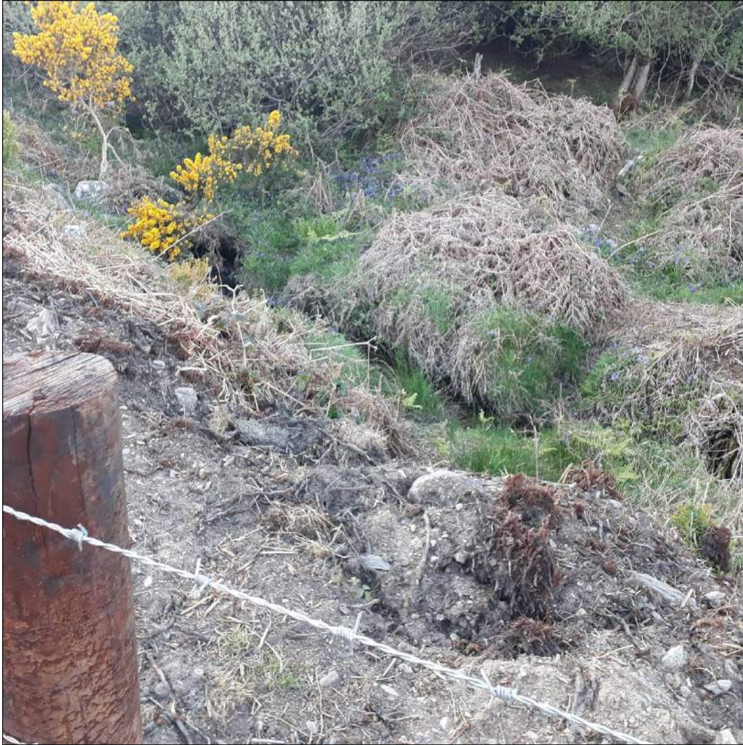
Earth movement and spreading of spoil in very close proximity to the watercourse with subsequent runoff and siltation risk.
