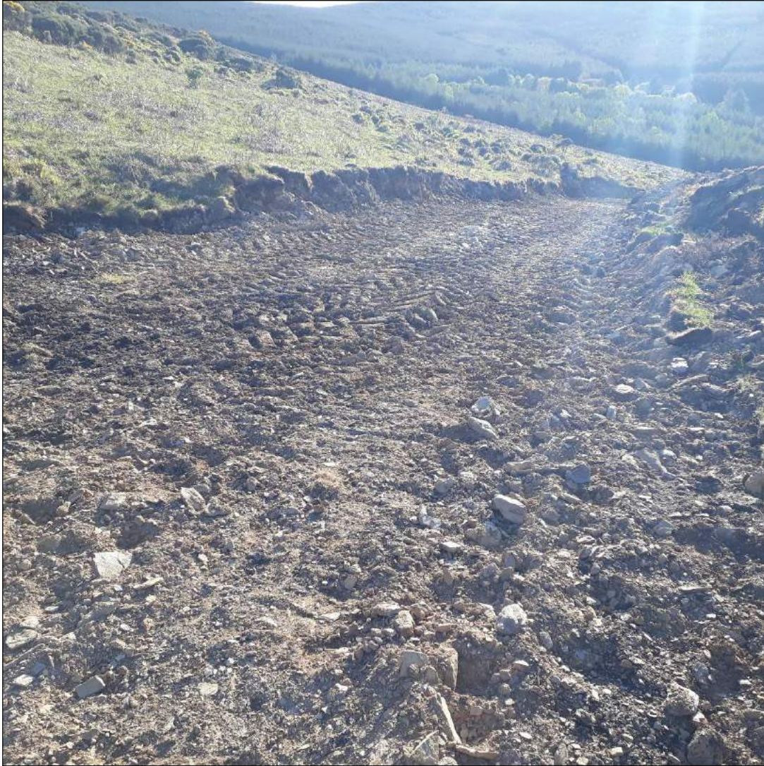
The steep slopes which the track has been developed on can be seen here. No water bars or other design features have been incorporated into the track to prevent gullying and significant erosion. The track leads downhill towards the Ballycumber Stream.
