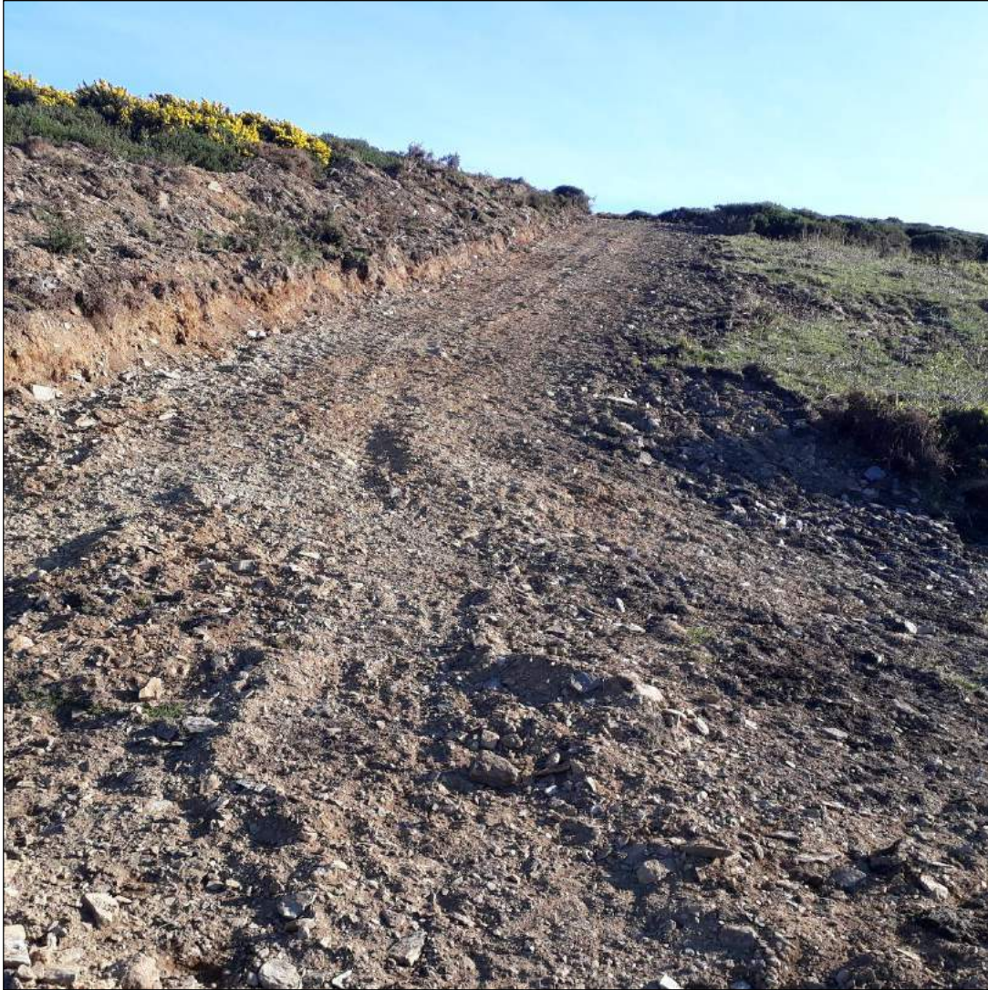
The track poses a serious runoff and erosion risk to the commonage.
