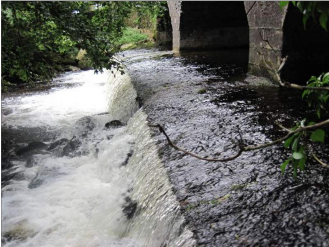
Ballinglen Bridge: This photo demonstrates the fish passage issues associated with laminar flow, flow velocity and the perching associated with this scour protection apron.
