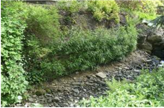
Example of willow spiling used in a river channel (Source: H. Dangerfield, Royal Haskoning.
