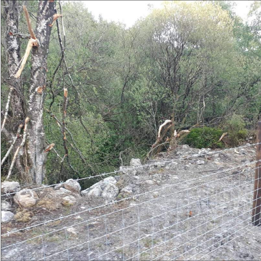
Spoil and excavated material has been pushed into the riparian zone with damage to mature trees and other vegetation.
