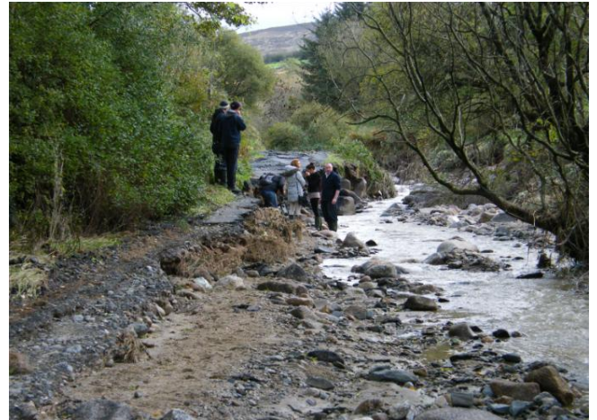
Road washed away in fluvial flooding.
